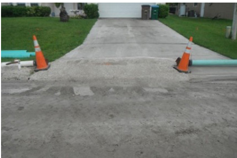
Dewatering Pipes
